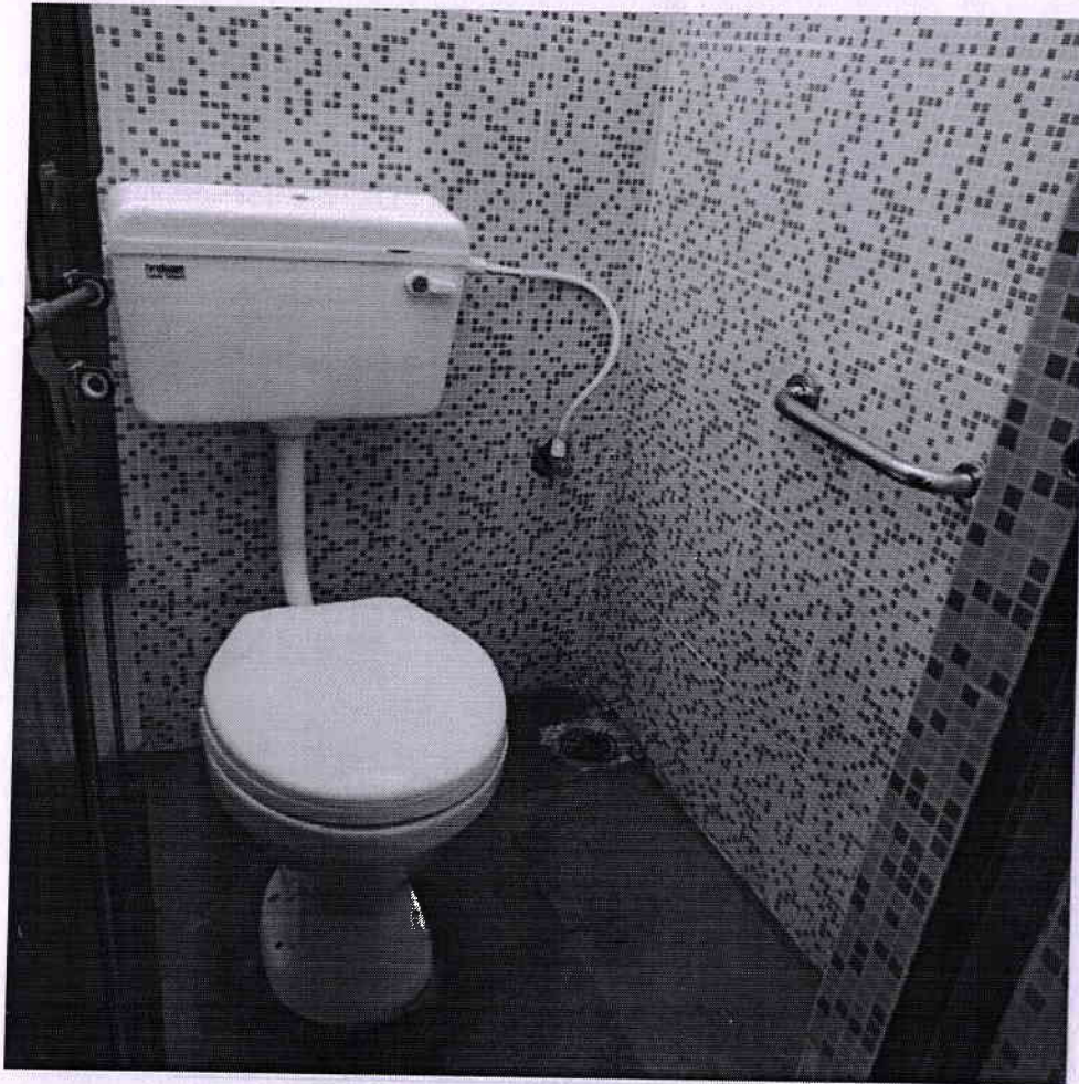
WASHROOM FOR PHYSICALLY CHALLENGED
